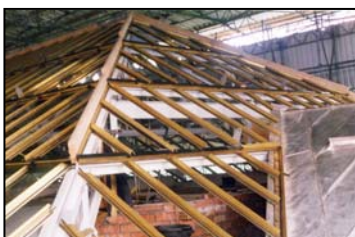
View of the structure of the brass roof, before covering.
