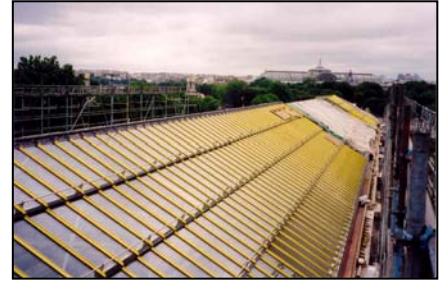
The brass roof during vitrifying
