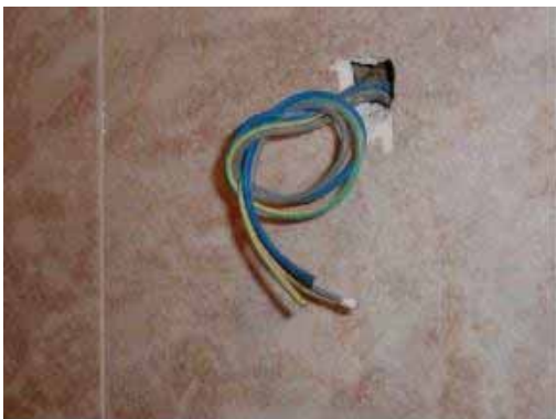
Figure 1 Typical safety hazards in residential installations: bare & live conductors, or overloaded sockets
