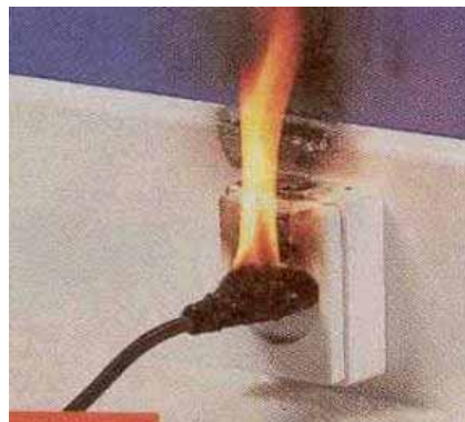
Figure 1 Typical safety hazards in residential installations: bare & live conductors, or overloaded sockets
